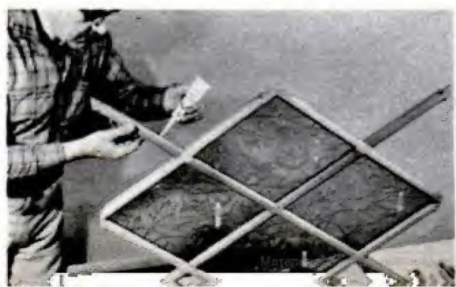
PLASTIC INSERTS are labeled for reassembly identity. GE Silicone Seal keeps the pieces from shifting
